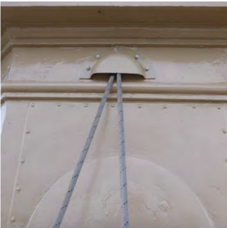
Figure 2. The painted copper cowl was screwed and caulked in place from the exterior.
