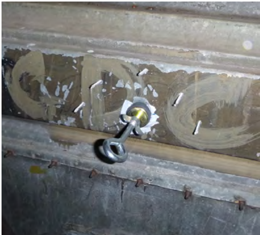
Figure 3. An expandable rubber plug was installed from the interior of the rigging hole
