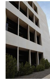
Figure C.17: Photo 3E - Precast Fin System
