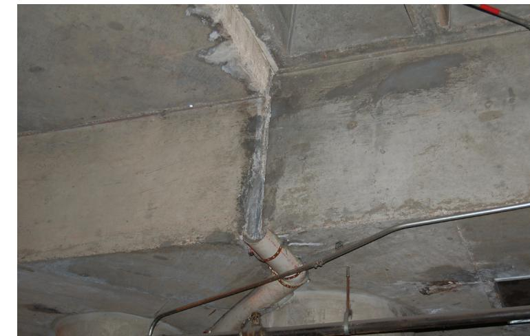
Figure C.33: Photo 5F - Expansion Joint in Garage
