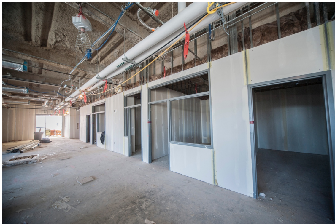
December 2017 – Herschler - 3 rd floor drywall installation
