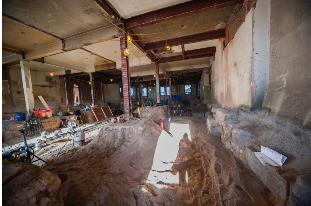
December 2017 – Garden Level West excavation for mechanical piping installation
