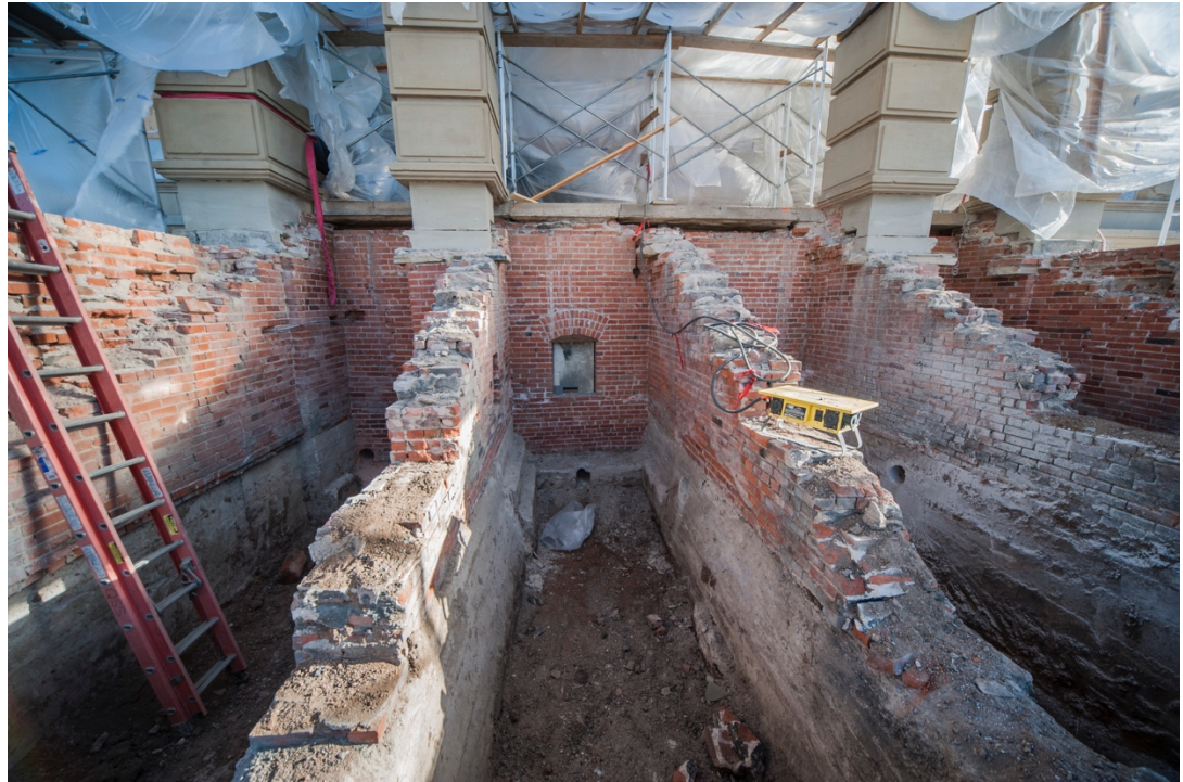
December 2017 – Capitol West Stairs repairs
