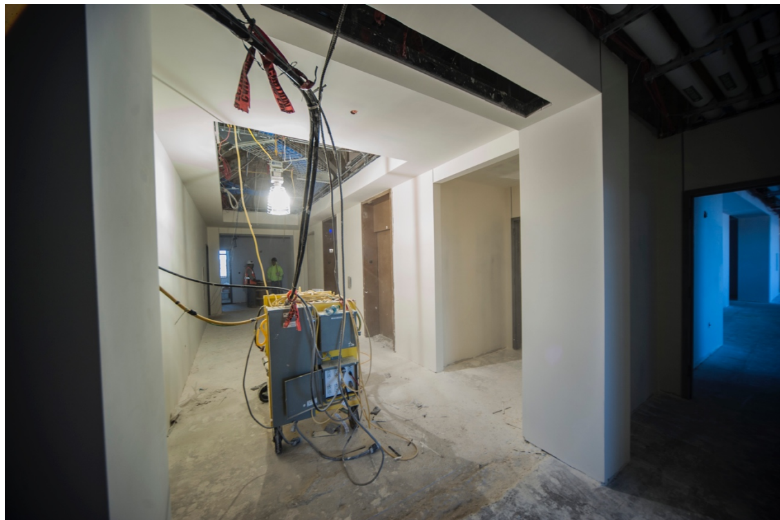
December 2017 – Herschler – 4 th floor drywall installation
