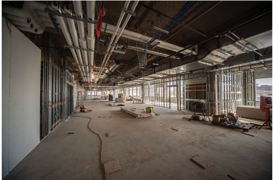
December 2017 – Herschler – 2 nd floor drywall installation
