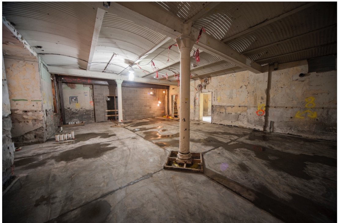
December 2017 – Garden Level East - Completion
