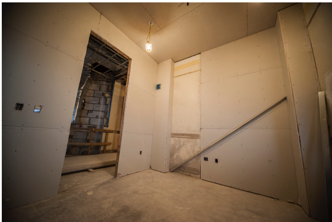
December 2017 – Capitol 3 rd floor drywall installation
