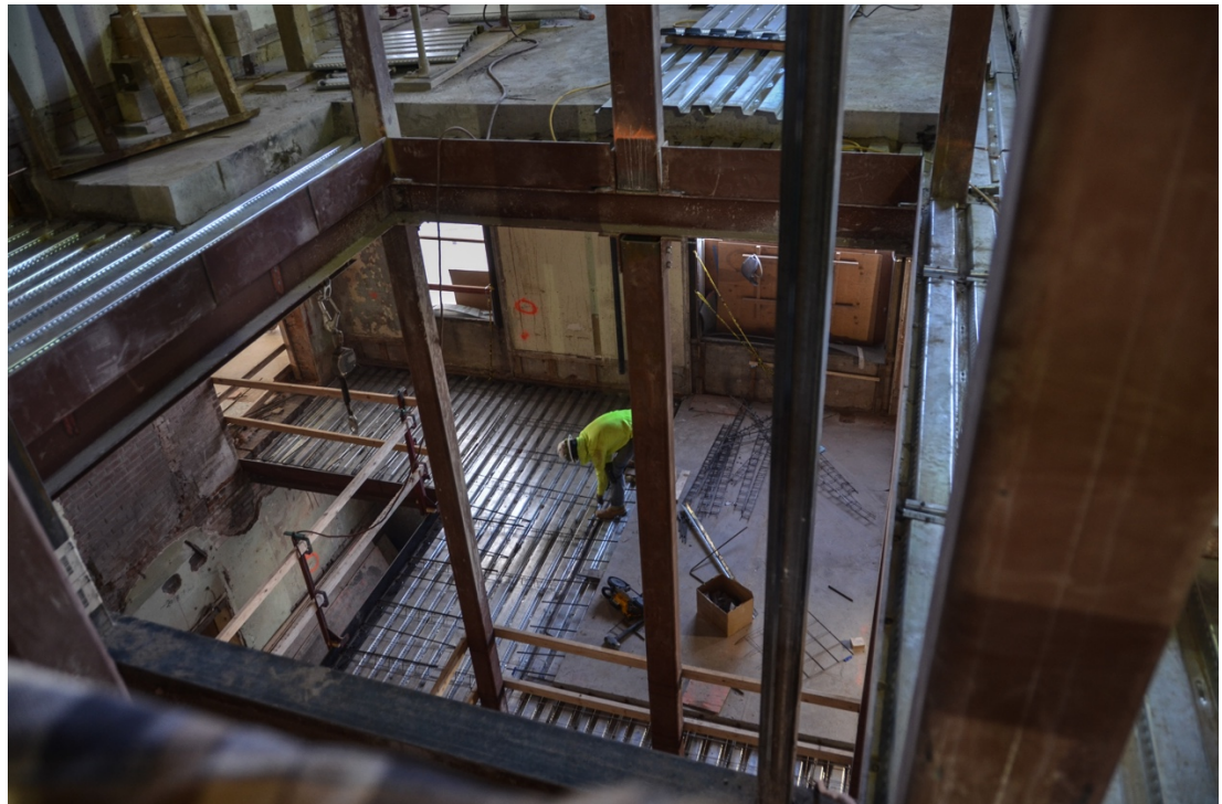
December 2017 – Capitol Elevator installation
