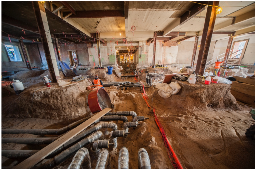
December 2017 – Garden Level West installation of mechanical piping
