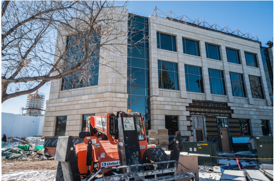
December 2017 – Herschler exterior stone installation
