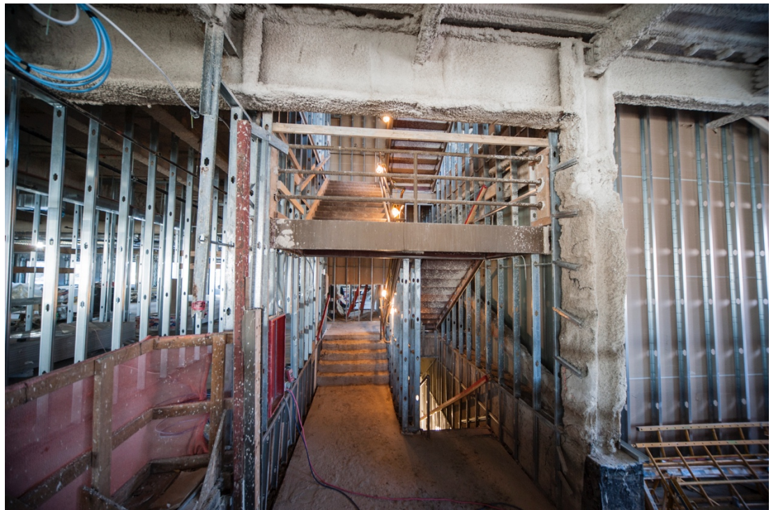
December 2017– Herschler – 1 st floor drywall installation
