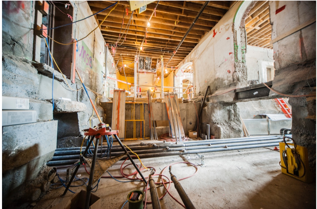
December 2017 – Garden Level West mechanical equipment installation
