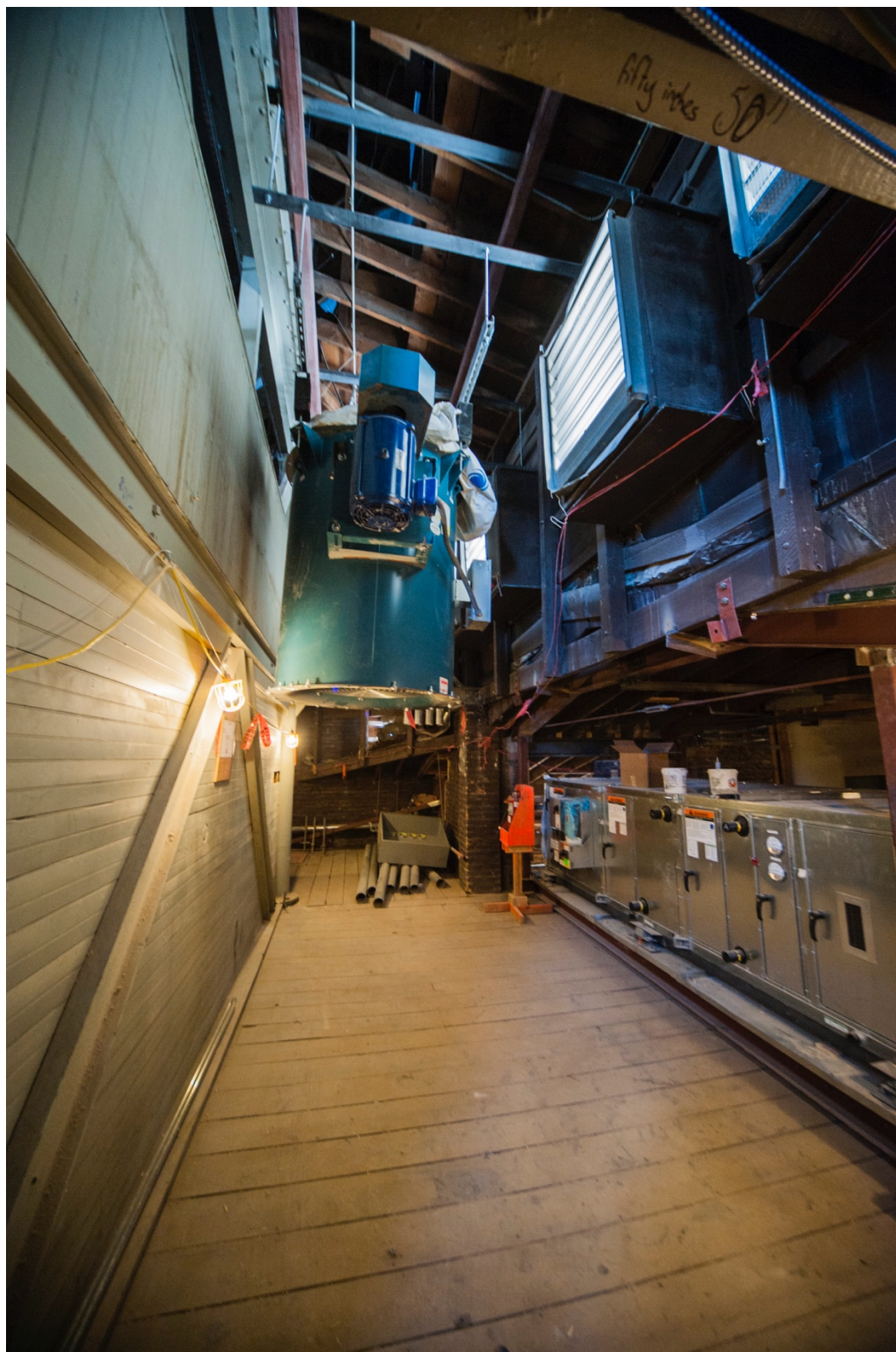
December 2017 – Capitol Attic
