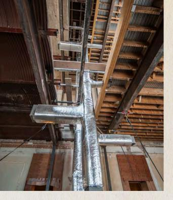
are efficiently organized and will be easier to maintain over time. New mechanical rooms have been located adjacent to the vertical chases on the garden level of the building to most effectively manage these building systems. These infrastructure cores are located on every floor of the building and also include public restrooms and new elevators. There are now six public women's restrooms and six public men's restrooms in the building.
