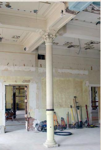
The removal of the suspended ceiling tiles revealed column capitals, coffered ceilings, crown moldings, picture rail, and decorative paint. The invasive work necessary to upgrade mechanical, electrical, and plumbing systems revealed these treasures and allowed the restoration of these historic features.
